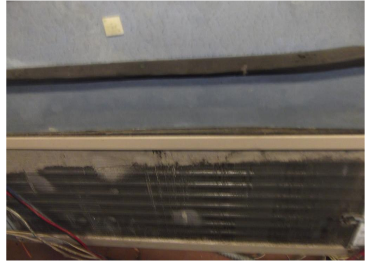
Room 117 PTAC Coil
