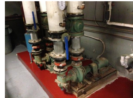
Heating hot water pumps
