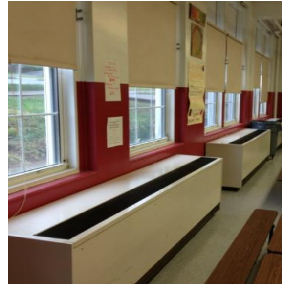
Unit ventilators serving cafeteria (3)
