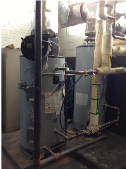
Natural gas fired domestic hot water heaters
