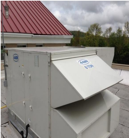
RTU#5 serving Media Center
