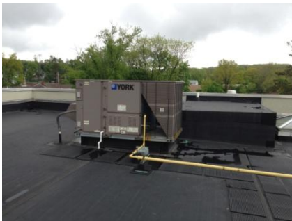
RTU#1 serving top floor class rooms
