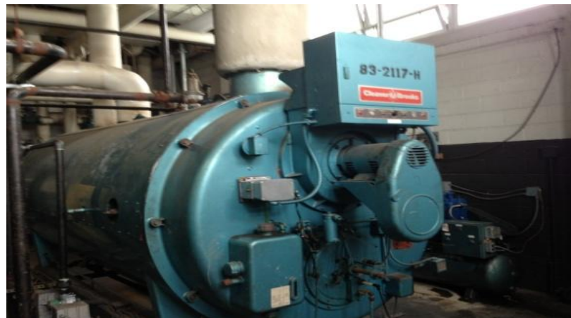
Fire tube heating hot water boiler
