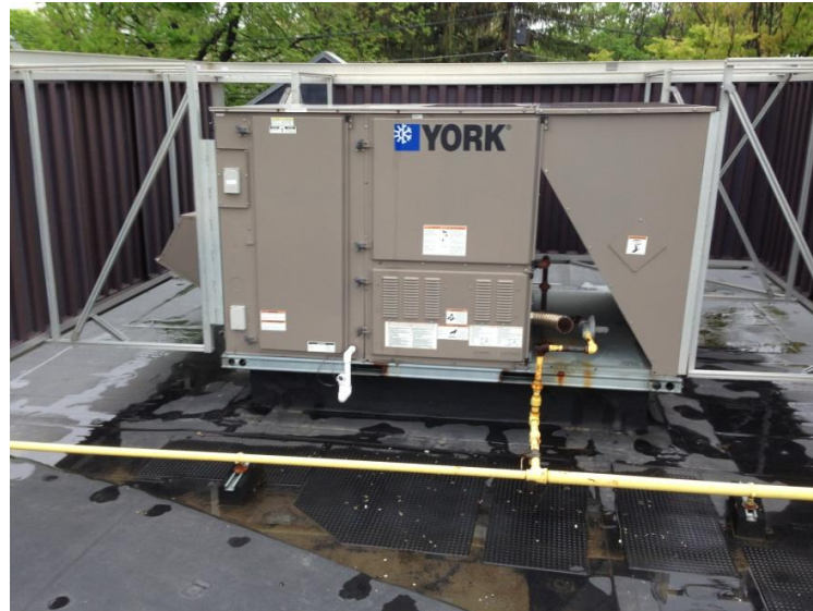
Rooftop unit serving the Media Center
