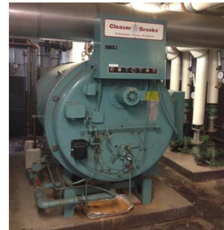
Fire tube heating hot water boiler
