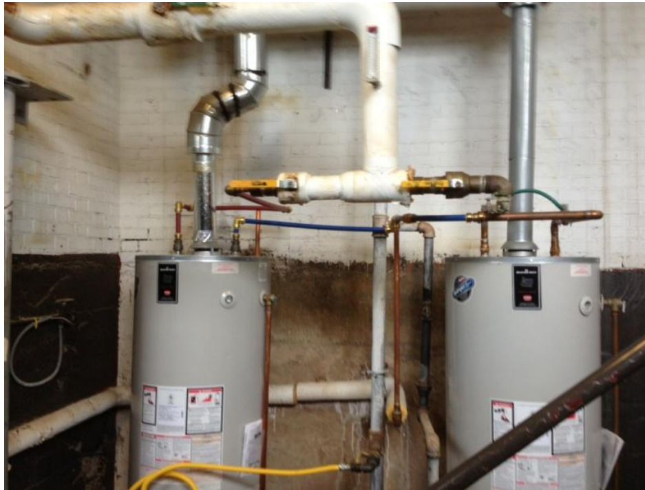
Natural gas fired domestic hot water heaters
