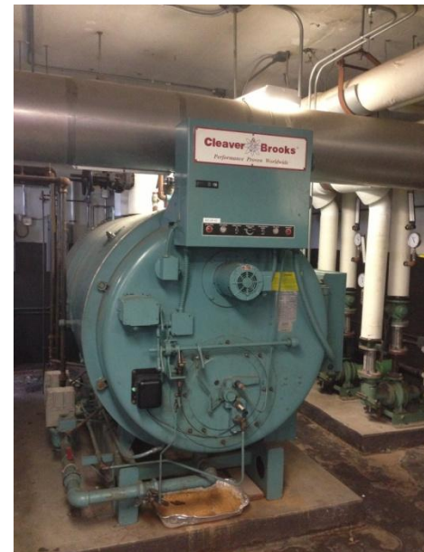
Forest E.S. Boiler
