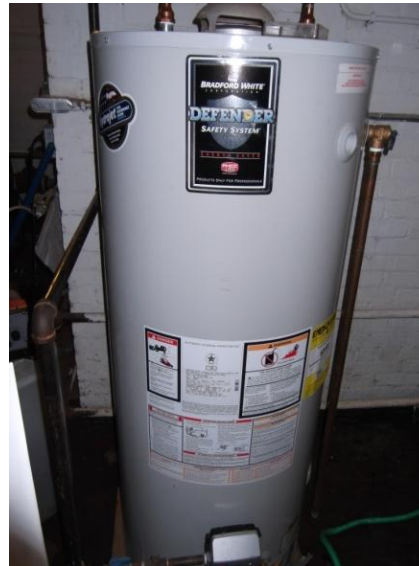
Domestic Water Heater
