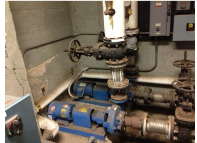
Heating hot water pumps for 1967 section of building
