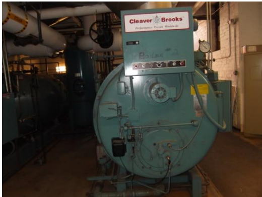
Fire tube steam boiler
