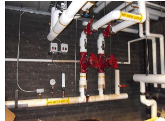
Heating hot water pumps
