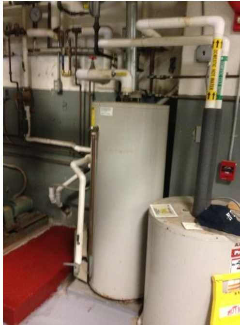
Gas-fired water heater (left) and electric water heater (right)
