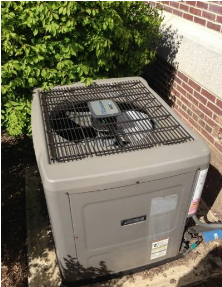
Condensing unit serving OT/PT
