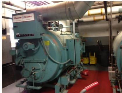
Fire tube hot water boiler
