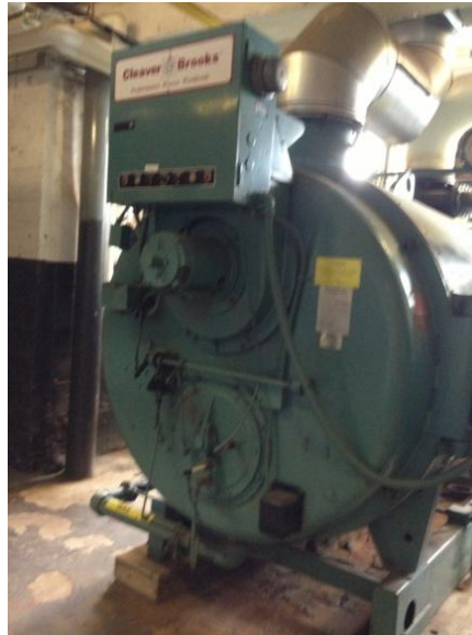
Fire tube steam boiler
