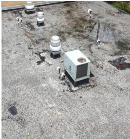
RTU serving main office
