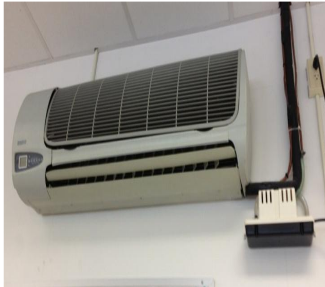
Ductless evaporator unit (typ.)
