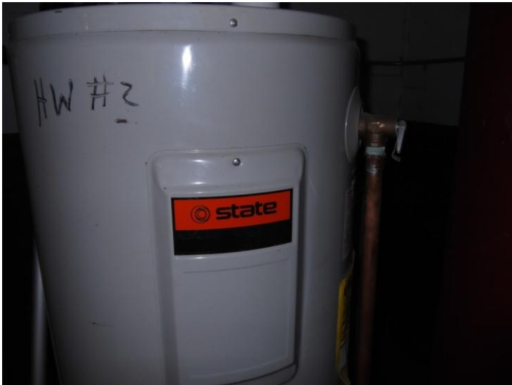
HW#2, Electric Water Heater
