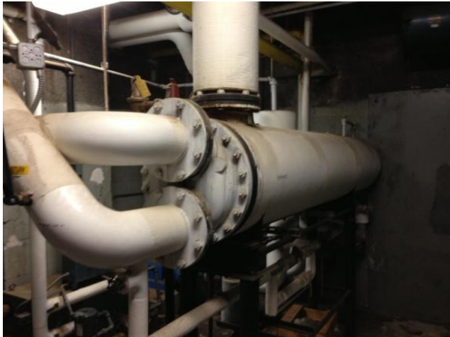
Steam to heating hot water heat exchanger (1 of 2)
