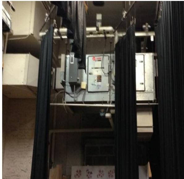
Auditorium AHU (1 of 2)
