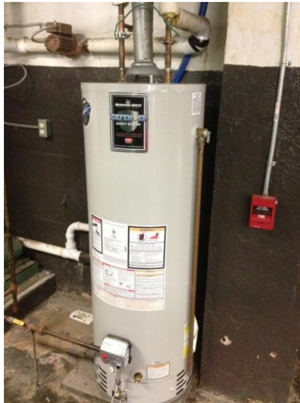
Domestic Water Heater
